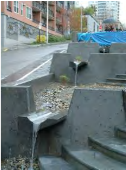
Figure 2.3: “Green Street” with Cistern Steps, Vine Street, Seattle
