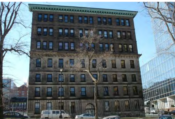
Figure 5.2: Dennis Building from Granville Street
