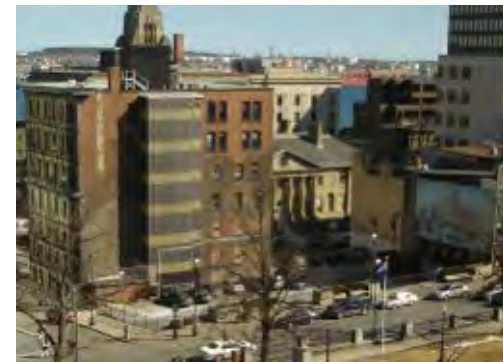
Figure 5.3: Birk's/Truscan Site from Barrington Street
