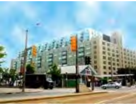
Figure 5.8: Example of new structure erected on existing building
