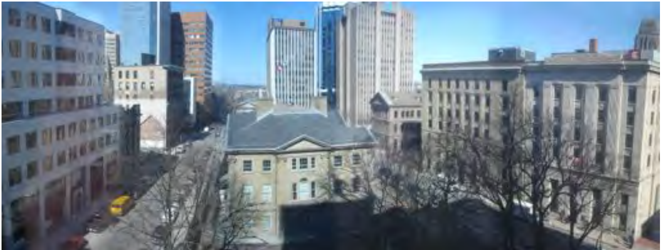
Figure 1.3: Province House and surrounding buildings
