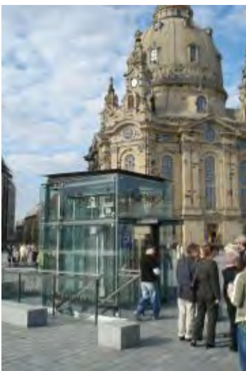
Figure 3.12: Contemporary kiosk/underground parking access placed in historic context
